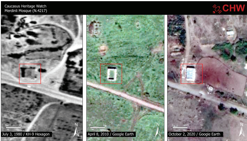
FIGURE 2.16. Satellite imagery of the Merdinli Mosque (N.4217) in Fuzuli. 1980 US reconnaissance imagery ( left ) shows the mosque intact (image source: USGS). Imagery from 2010 ( middle ) shows the roof has been removed (image source: ESRI, © 2010 Maxar Technologies). A subsequent October 2020 image ( right ) shows the mosque has been roofed and an adjacent enclosure constructed to the east consistent with reuse as an animal pen (image source: Google, © 2025 Maxar Technologies). © Caucasus Heritage Watch 2025.
