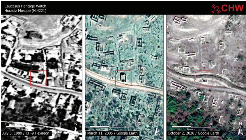
FIGURE 3.5. Categorical threshold of detectability. Horadiz Mosque (N.4221) seen intact in a 1980 HEXAGON image ( left ) was damaged by 2005, by which time its roof had been removed ( middle ) (image source: USGS). Between 2005 and 2010, a trench was cut that removed the northern half of the structure leaving only the south wall and portions of the east and west walls still standing at the time of the 2020 image ( right ) (image source: Google, © 2020 Maxar Technologies). © Caucasus Heritage Watch 2025.
